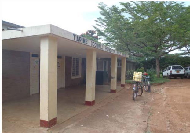
Tarime Goodwill Foundation Hospital
